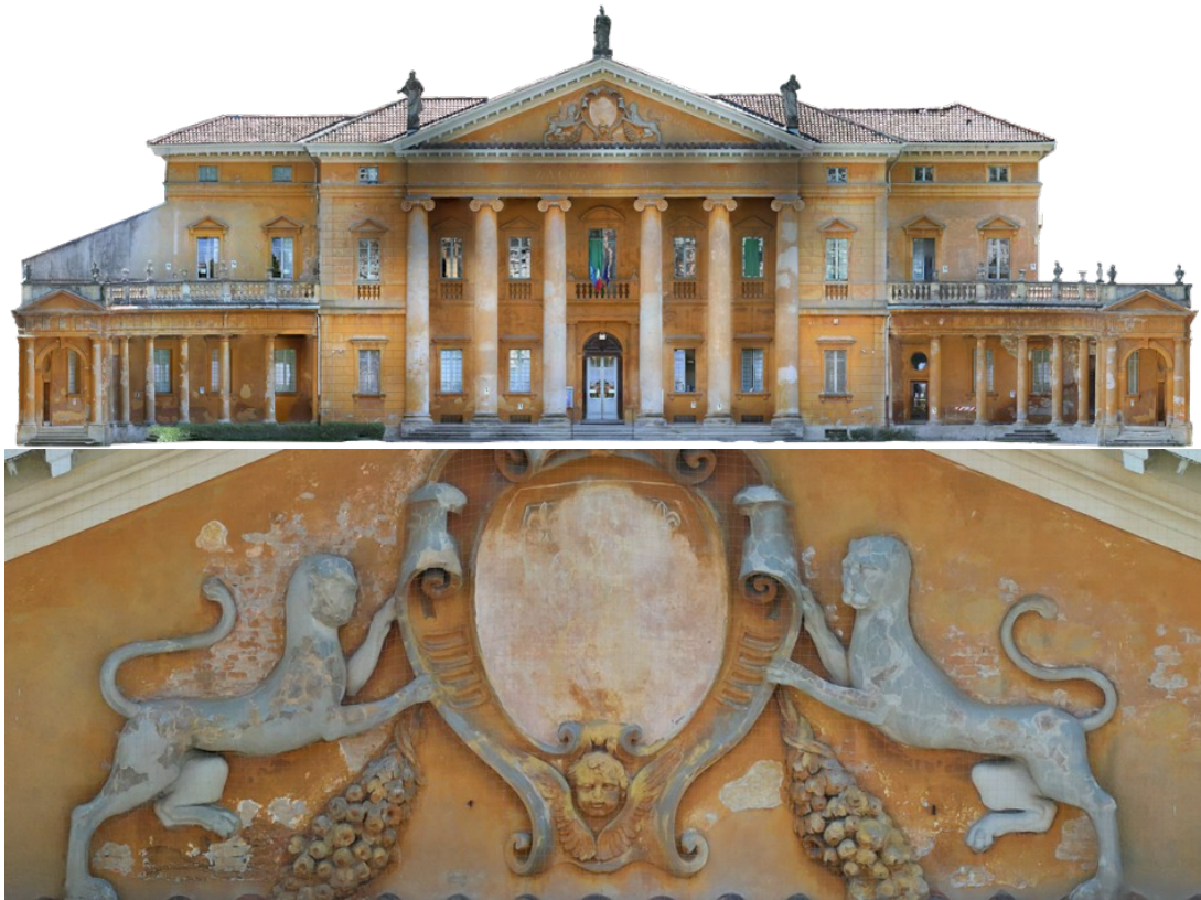
Figure 70. Hi-res orthophoto of the façade from photogrammetry (top) and an illustrative detail (bottom)
