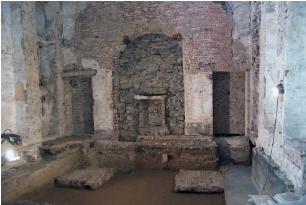
Figure 42. Excavations of the west choir revealed two foundation stones
